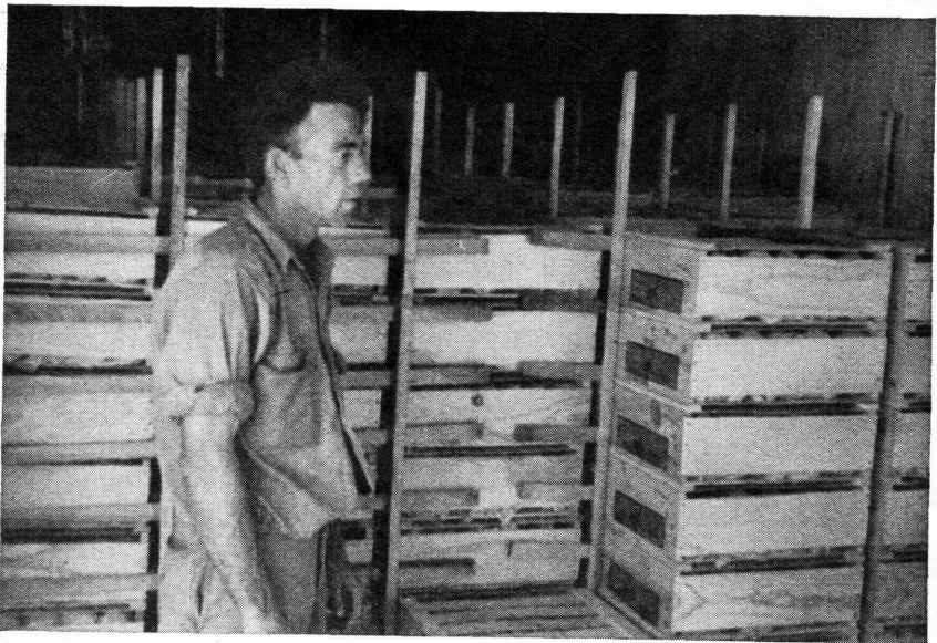
FIGURE 20.—Western boxes being loaded in a refrigerator car with the longest dimension of the boxes crosswise in the car. Note the vertical corner bracing.
